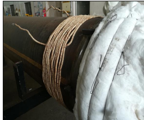
Fig. 4: Post Weld Heat Treatment Process.
