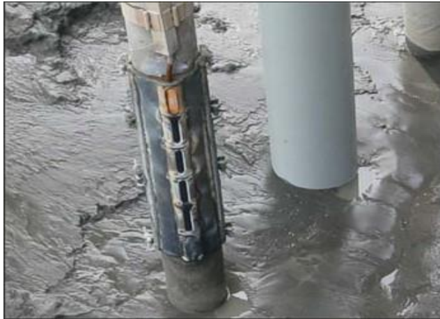
Fig 3. a: Alduco : Offshore Corrosion Control [7]
